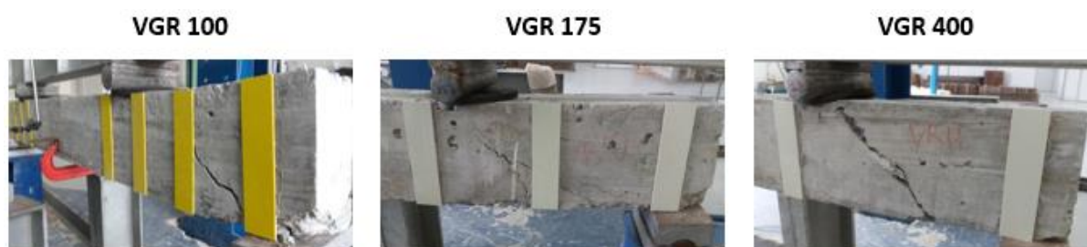
Figure 7: Rupture of beams of groups: a) VGR 100; b) VGR 175 and c) VGR 400
