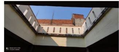
Upside View from the first floor
