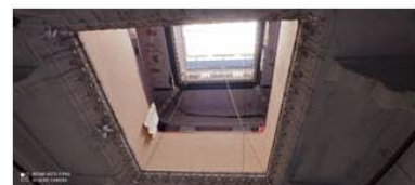
View from the ground floor
