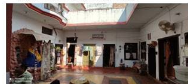
View of northern wall
