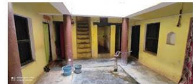
View of northern wall
