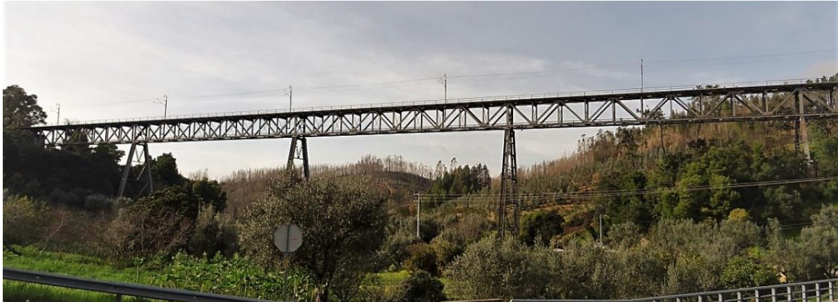
Figure 7: General view of the bridge under study
